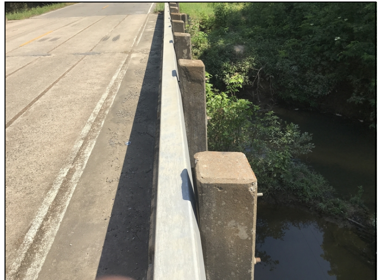
Right rail is loose with sheared bolts at Span 1 & 2.
