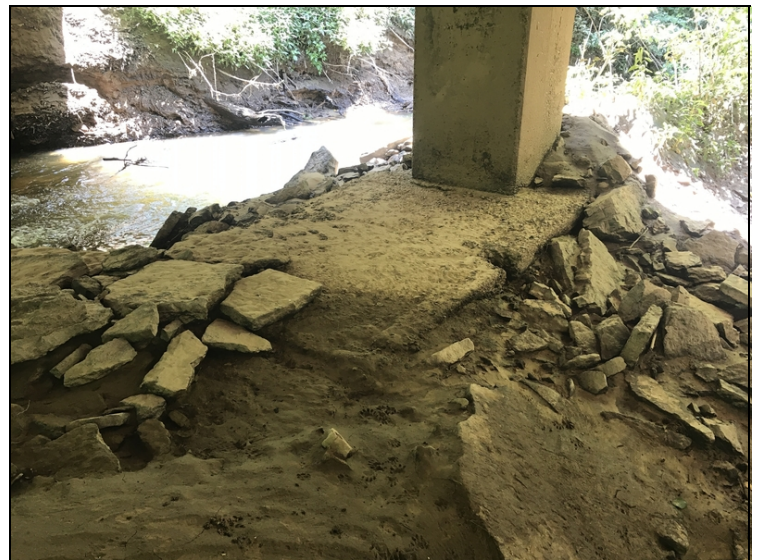
Footing exposed at Bent 1.
