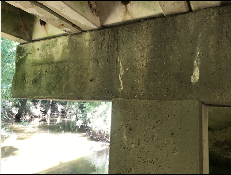
Cracks & spalls to cap at Bent 1.
