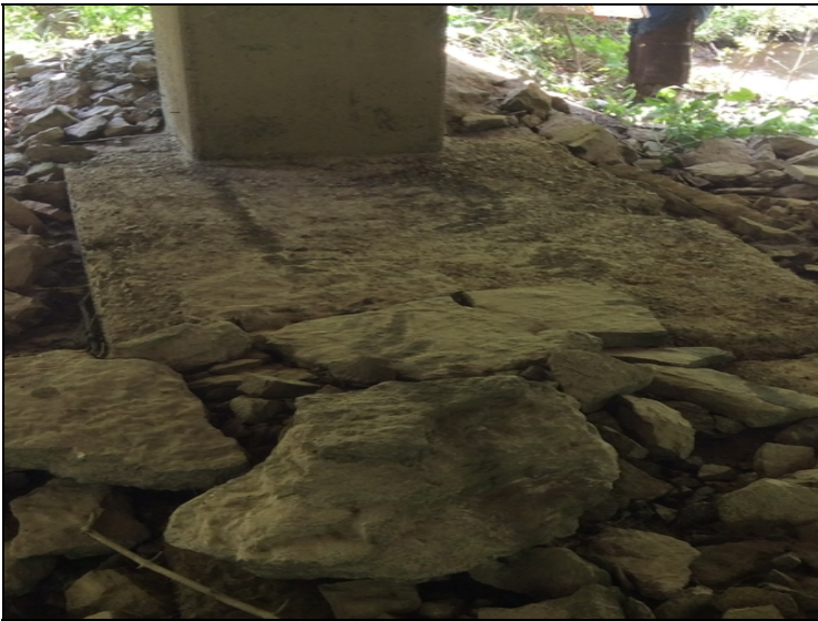
Footing exposed at Bent 1.
