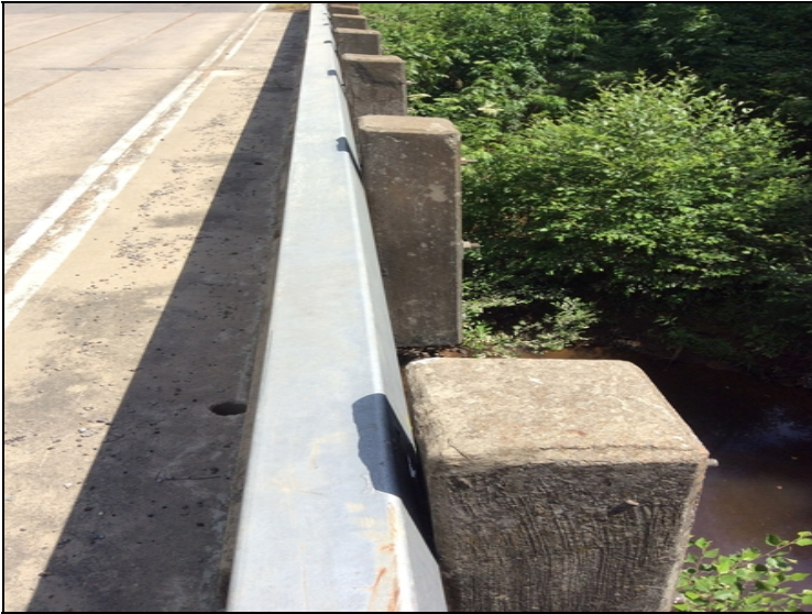
Right guardrail is loose with sheared bolts at Span 1 & 2.
