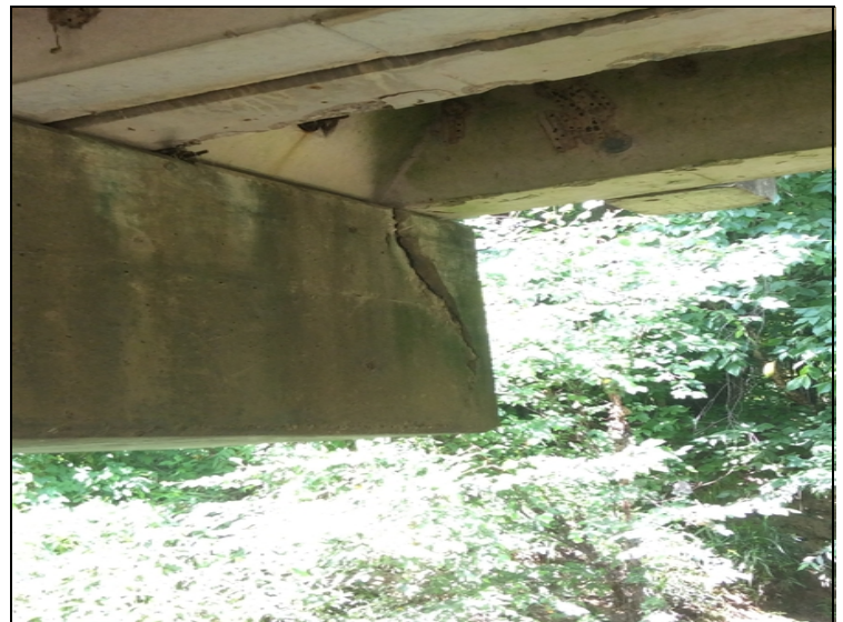
Cracks & spalls to cap at Bent 1.
